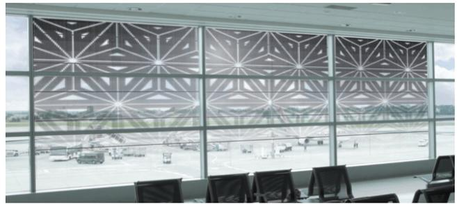
Figure 1: Transparent screens installed in the Rotterdam The Hague Airport, displaying geometric figures and reducing the incoming sunlight. Courtesy of VideowindW [3].
