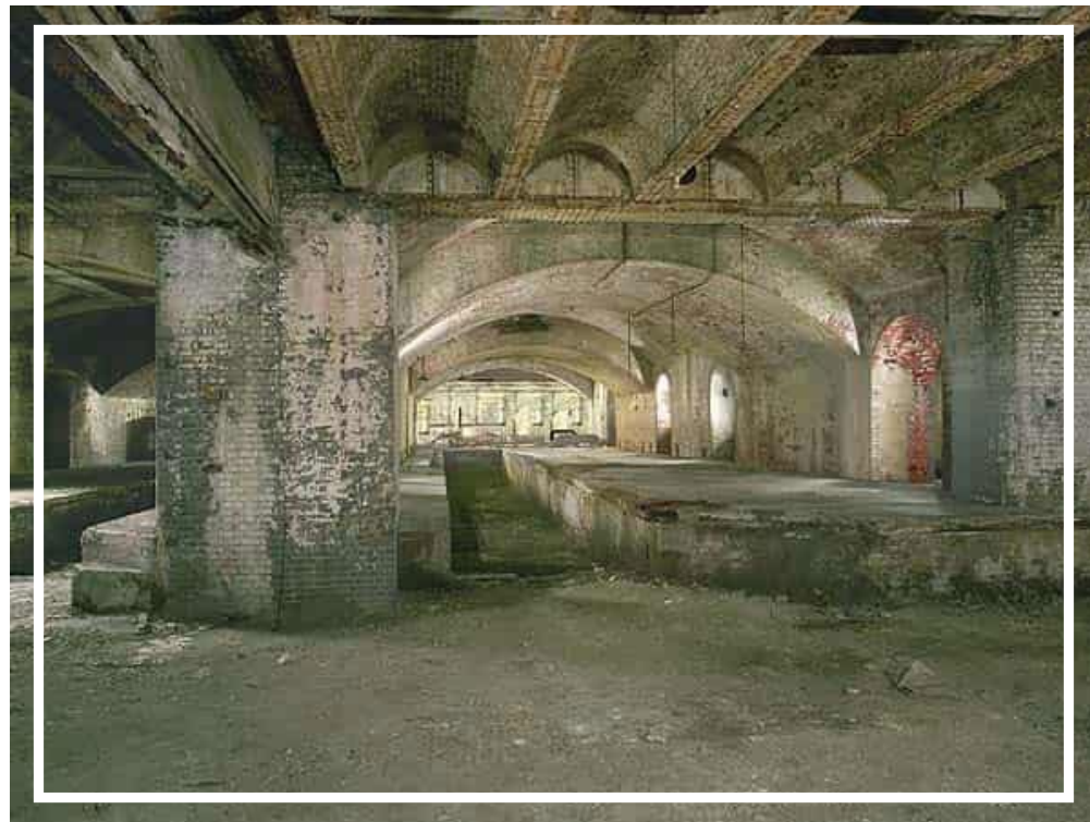
Lower rail level, between Shoreditch High Street and Wheeler Street (Braithwaite Street)
