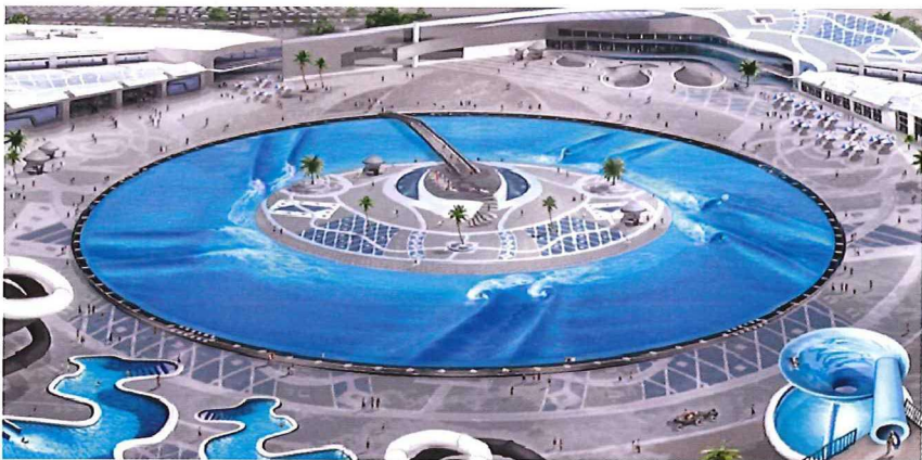
Figure 1-5. Artist's impression of the wave pool for a water park complex (reproduced with permission of Liquid Time Pty Ltd). The pressure sources are travelling anticlockwise, generating left-handed waves.
