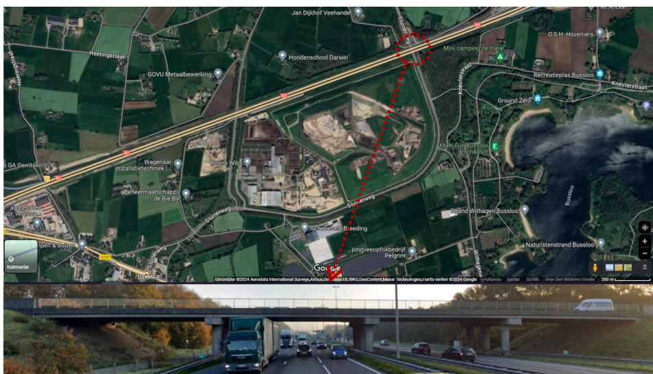
Fig. 3. Sluinerweg viaduct: In-situ pilot project.
