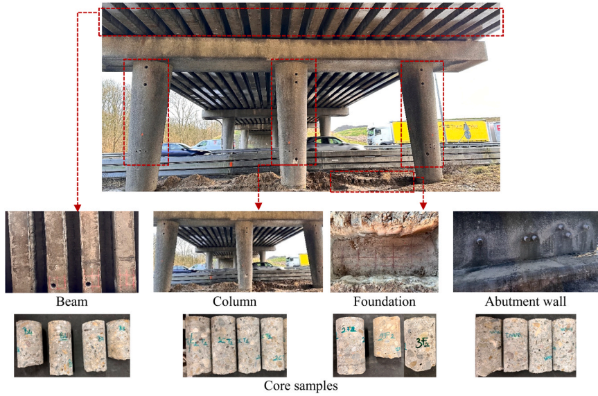
Fig. 4. Side view of the Sluinerweg viaduct (top), test locations (middle) and core samples (bottom).
