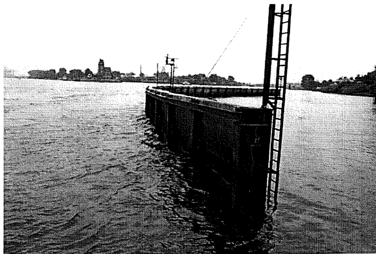
Figure 1.1. The prototype Current Deflecting Wall in the Köhlfleet harbour in Hamburg (C. Kuijper)
