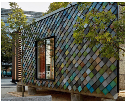
Fig. 36 - Pretty Plastic facade, using the 'First one' tiles (source: Pretty Plastic, n.d.)
