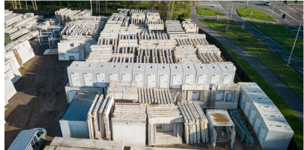
Fig. 4 - The temporary courthouse of Amsterdam was fully deconstructed and rebuilt at a different location (Cepezed)
