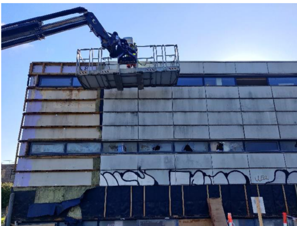
Fig. 17 - Dismantling of metal façade panels (Andersen et al., 2022)
