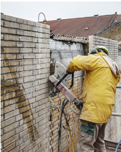
Fig. 19 - Reusing entire slabs of reused bricks (Lendager, 2019)
