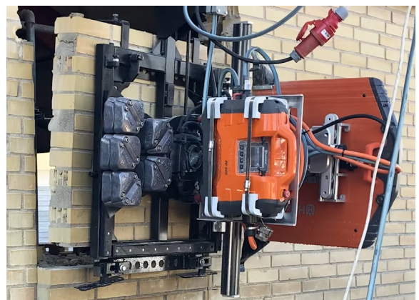
Fig. 43 - System to recover the bricks from donor building (Reconstructing The World, 2024)
