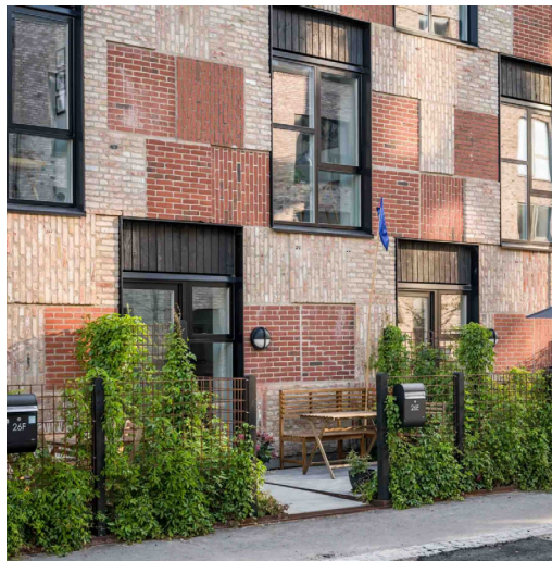
Fig. 19 - Reusing entire slabs of reused bricks (Lendager, 2019)
