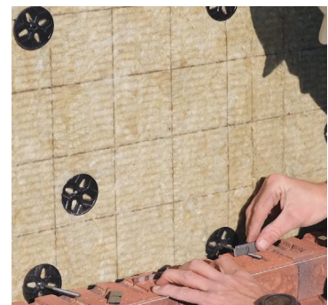
Fig. 21 - ClickBrick system (Wienerberger, 2025)
