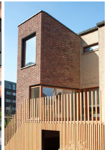
Fig. 20 - Reusing separated bricks (Rotor vzw/asbl, 2021)
