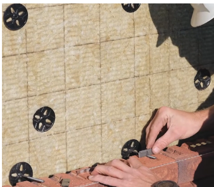
Fig. 40 - Connecting ClickBricks to the bearing wall (Wienerberger, 2025)
