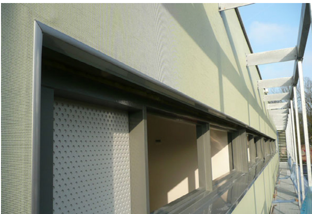
Fig. 29 - Examples with facade fabric cladding (source: Buitink-Technology, n.d.)
