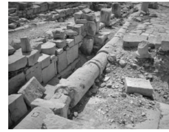
Stone conduit in Amathus (sculptured stone water pipeline) with a small aperture used as an inspection hole covered by a flat stone and sealed with time mortar.
