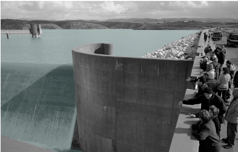
People gathered to observe the dam's water overflows.
