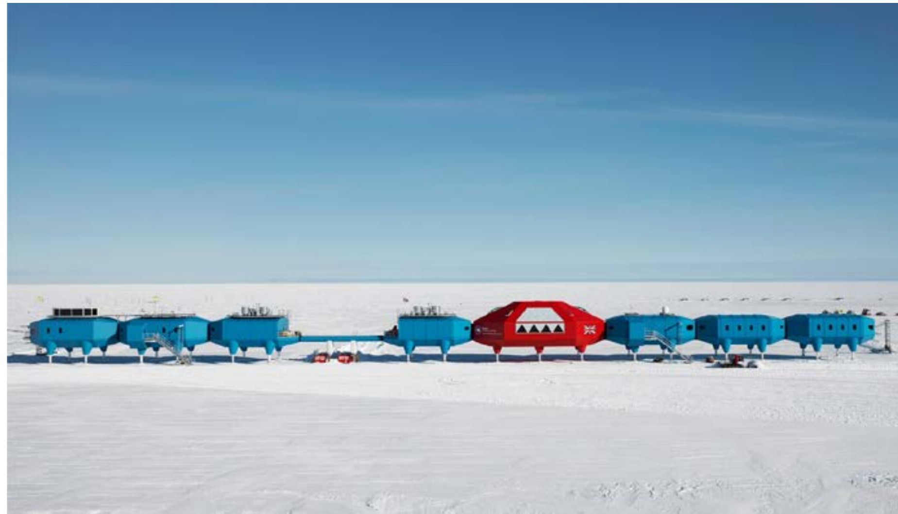
Halley VI - Antarctica research station Hugh Broughton Architects
