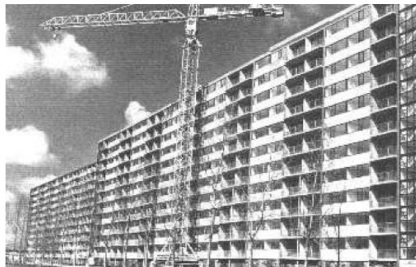
Figure 2.11 – Middelburg apartment building before the disassembling (Kristinsson, Hendriks, Kowalczyk, & te Dorsthorst, 2001)
