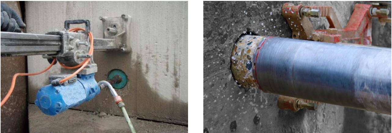
Figure 5.8 – Drilling procedure of sleeve holes (Rafa Adventure, s.d.) (Adamas homepage, s.d.)
