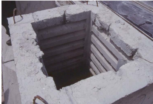
Figure 5.31 – A column pocket ready to host a column (FIB, 2008)
