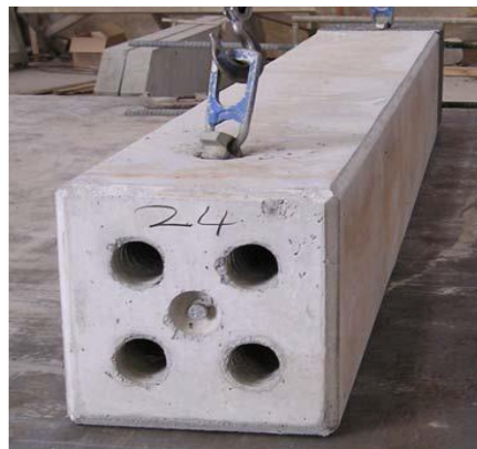
Figure 5.7 – Coupling sleeves in a column end (FIB, 2008)
