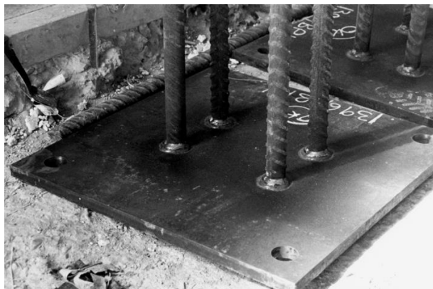
Figure 5.19 – Steel plate with pre-welded bars (FIB, 2008)
