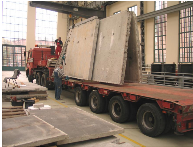
Figure 2.4 – Securing of second-hand slabs before their transportation (Asam C. , 2006)
