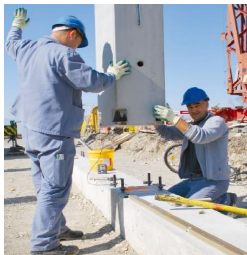
Figure 5.16 – Workers installing a precast column with column shoes (Circulariteit, 2018)
