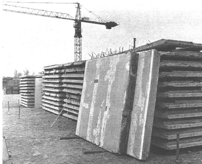
Figure 2.5 – Storage of second-hand slabs (Kristinsson, Hendriks, Kowalczyk, & te Dorsthorst, 2001)
