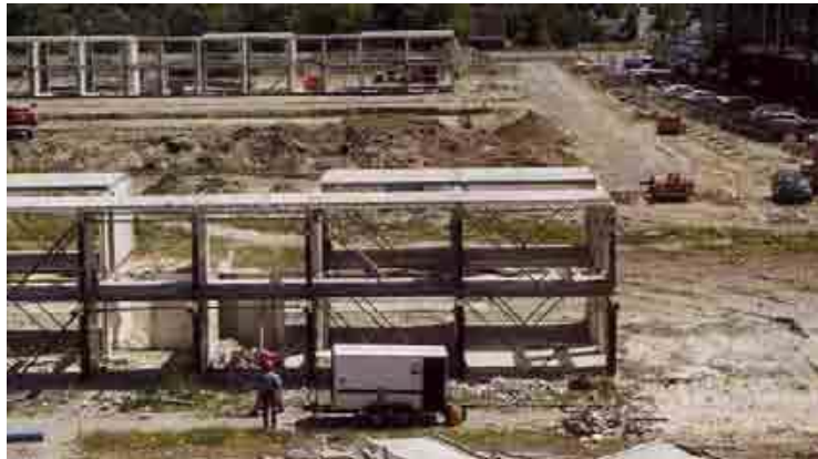
Figure 2.12 - The main structure after removing the upper floors (Naber, 2012)
