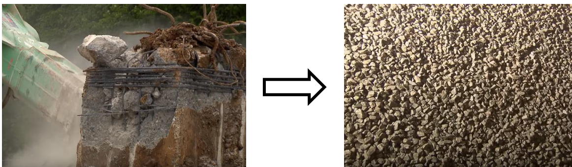
Figure 1.3 – Demolition process to gravel (Recycling concrete)
