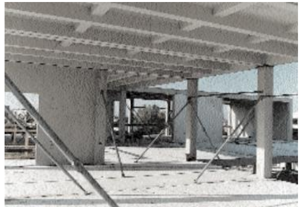
Figure 2.9 – Moducon 2000 on-site mounting and overall view (Bouwsystemen in de scholenbouw: Moducon-2000, 1999)
