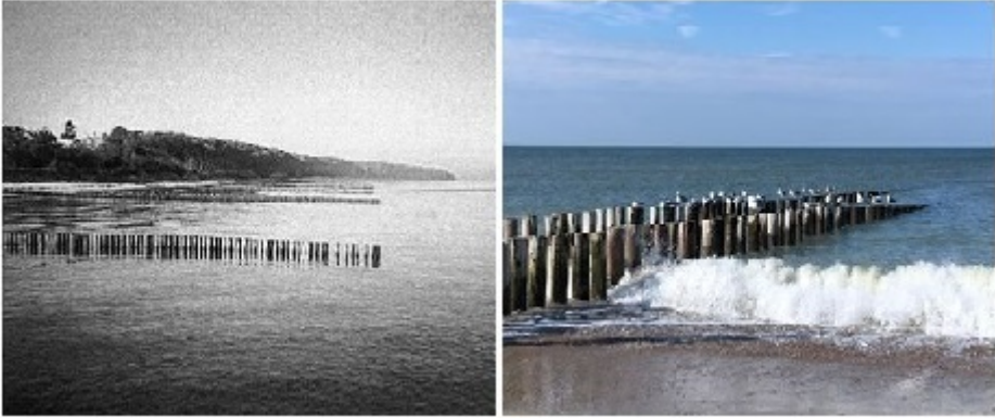
Figure 2.1: Left: The single row permeable pile groins at the southern coast of the Baltic sea, German [Raudkivi and Dette, 2002] Right: The two-row permeable pile groin at Domburg coast, the Netherlands.
