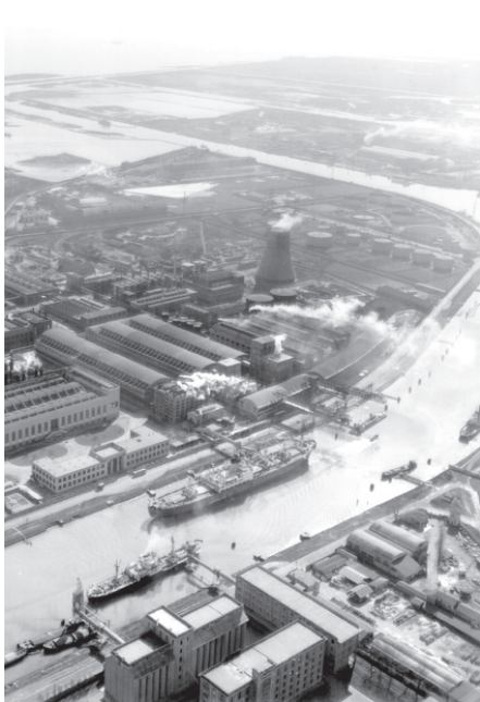
fig. 05/20 MONTECATINI EDISON, VETROCOKE PLANT AERIAL VIEW, 1967 - Source: lombardiabeniculturali.it
