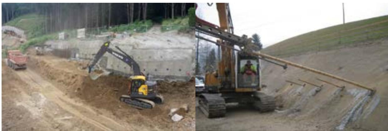
a) Standard soil nailing system
