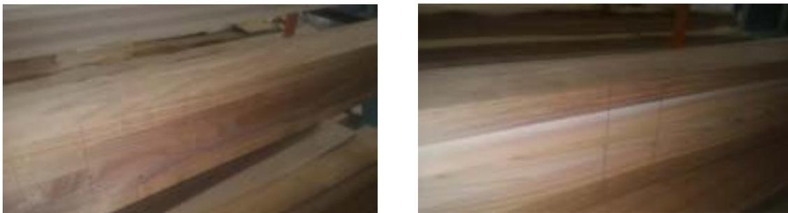
Figure 5: Blackwood glulam beam (left) and mixed glulam beam made with Blackwood and Sugi (right).
