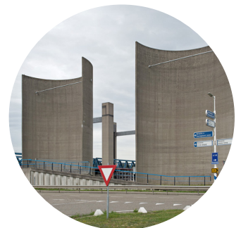
6. Calandbrug Windshield and noise barrier installations that are designed as a land art project
