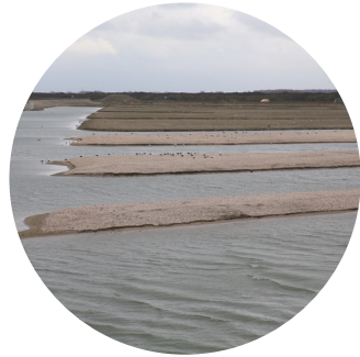
1. Vogelvallei The Port of Rotterdam Authority has redeveloped Maasvlakte's bird valley (The Vogelvallei), a nature reserve for birds, and enlarged it to 21 hectares. This redevelopment took place in close consultation with Bureau Stadsnatuur (Rotterdam's urban nature agency), H+N+S Landscape architects and various nature organisations.
