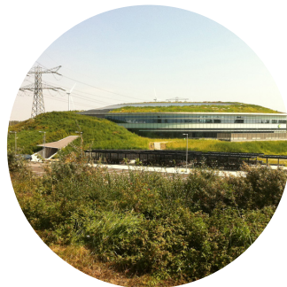
4. BP Refinery office building Built into an artificial dune, not just to mimic the nearby environment, but also to create a safe environment for the offices
