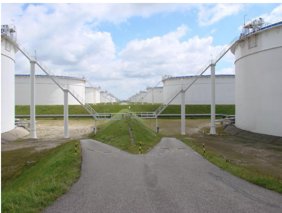
Current state of petrochemical storages
