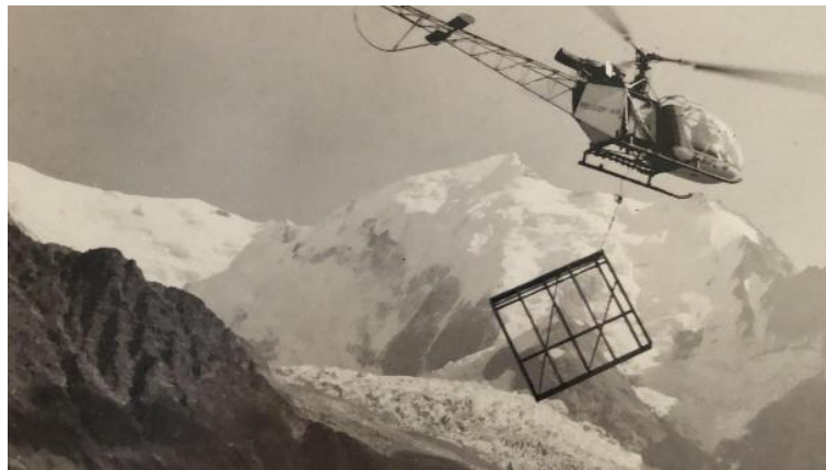
Figure 9. Reconstruction of refuge des Grands Mulets by helicopter, massif du Mont-Blanc, E. Dessert, 1960.
