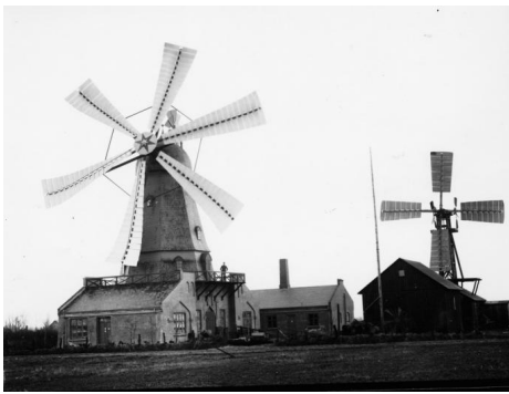
Figure 1.1: la Cour's experimental turbines at Askov, Denmark, as they stood in 1897. Source: Vejen Lokalhistoriske Arkiv.
