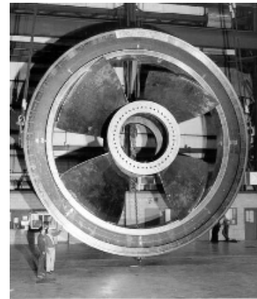
Figure 4.2 Straflo turbine (Andritz group)
