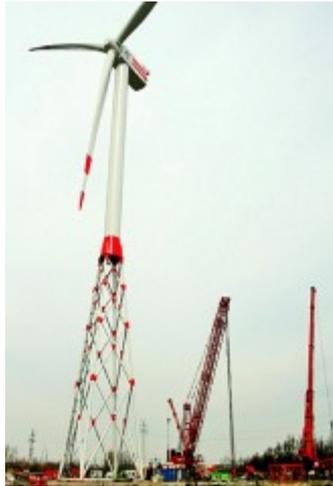
Figure 2.5 REpower 5MW Wind Turbine on a Jacket Substructure [11]
