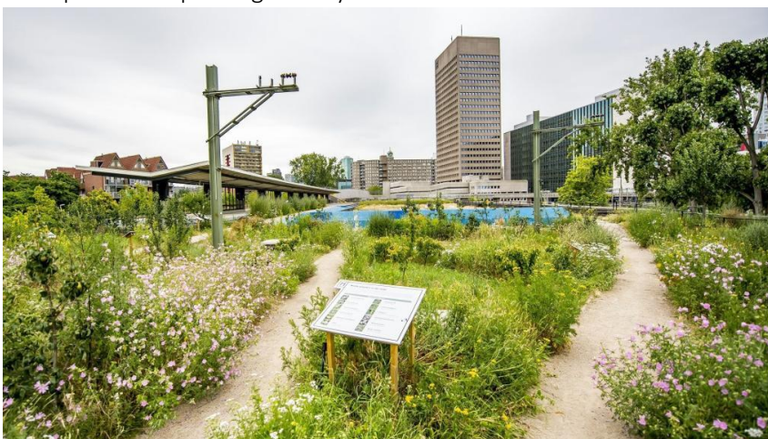
Figure 3: Public green roof Rotterdam (Gemeente Rotterdam, 2019)
