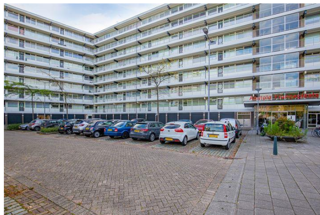
Figure 2: Gallery flats in Ommoord (Funda, n.d.)
