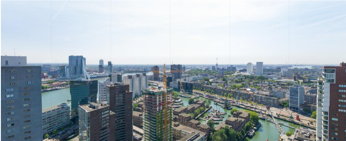
Figure 29: South-west view at 120m from the location of the Cooltower (Cooltower, n.d.)
