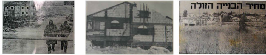
FIG. 3.38 Nirit under construction – Brought in (Pinhas, 1987); (Yedioth Ahronot, 1987); (Glick, 1988)
