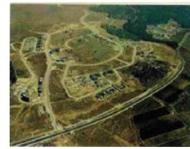
FIG. 5.36 Construction of Phase 1, 1997. (Ela'ad Council)
