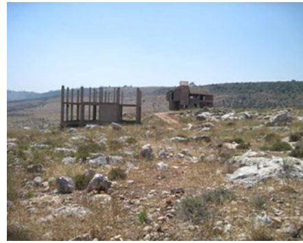
FIG. 3.46 Uncompleted buildings in the site of Ya'arit, 2014
