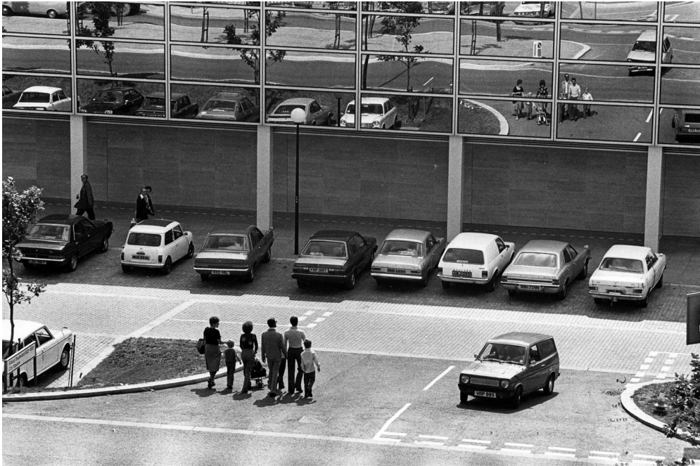
Figure 9. Exterior view of Milton Keynes' shopping centre, showing the mirror glass panels applied to the façade.
