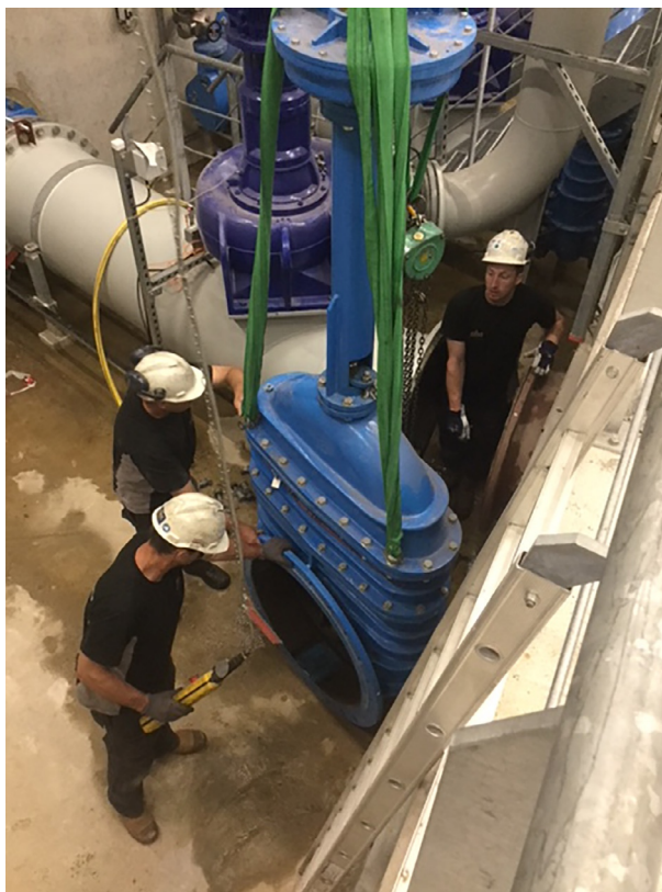
Fig. 4 Expanding the valve casing at Ramspol Barrier. (Image: Courtesy of Rijkswaterstaat, Tycho Busnach.)
