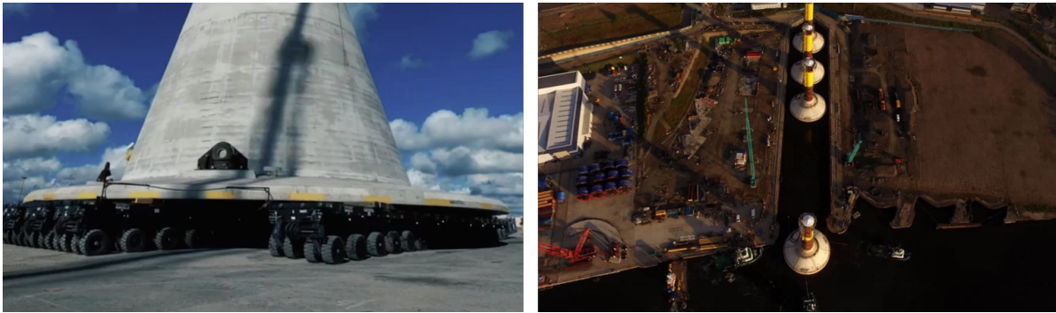
Figure 2.8: Load-out of GBFs from quayside (left) and dry dock (right) [39].
