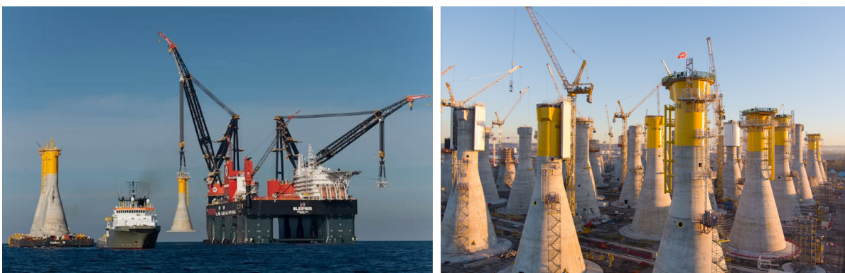
Figure 2.1: Installation (left) and construction quay (right) of the Fécamp OWF GBFs.
