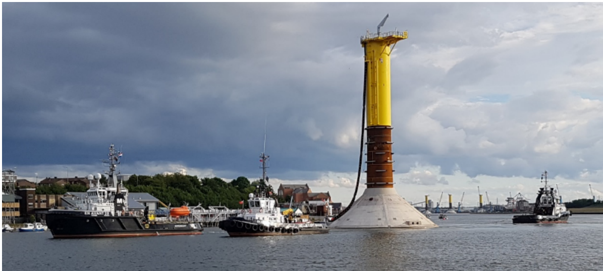
Figure 2.2: BOD self-buoyant GBF being towed out at River Tyne, Newcastle, UK [39].
