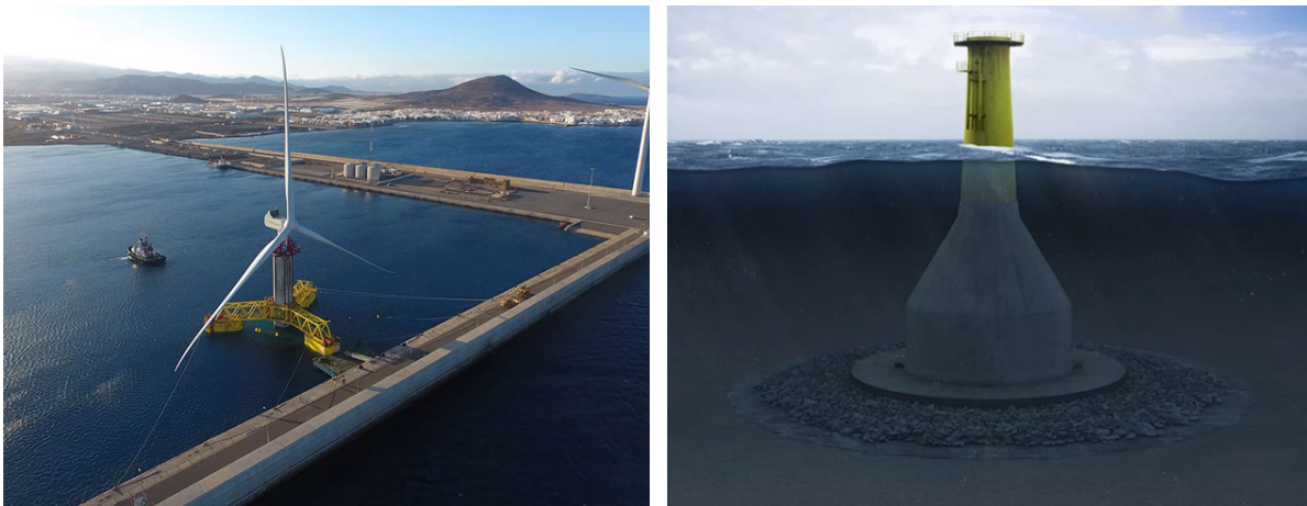
Figure B.3: ELISA/ELICAN concept by Esteyco (left) [23]. Cranefree concept in its final installed position (right) [5].
