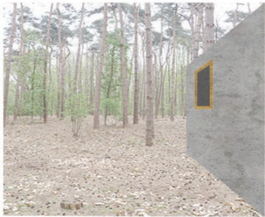
rough exposed concrete walls brass elements leaving stains
