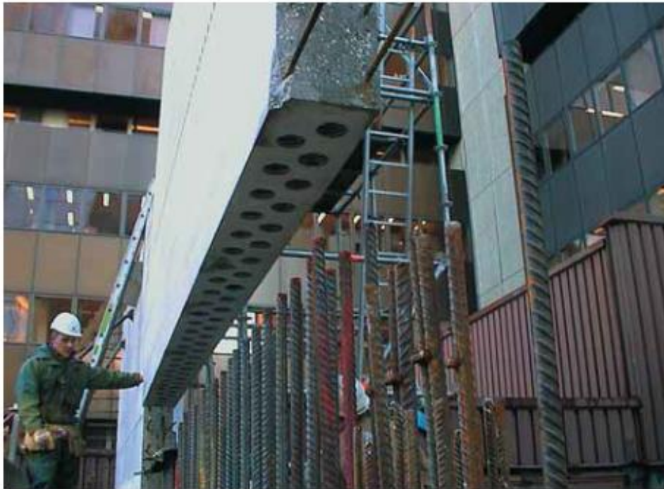
Figure 59 Placing of an element on starter bars [Bennenk]
