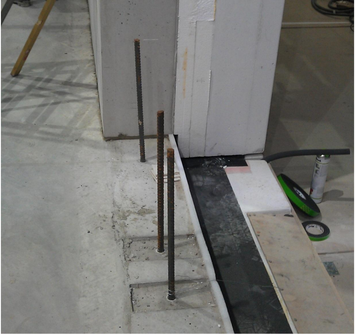
Figure 61 Elastic strip at a joint
