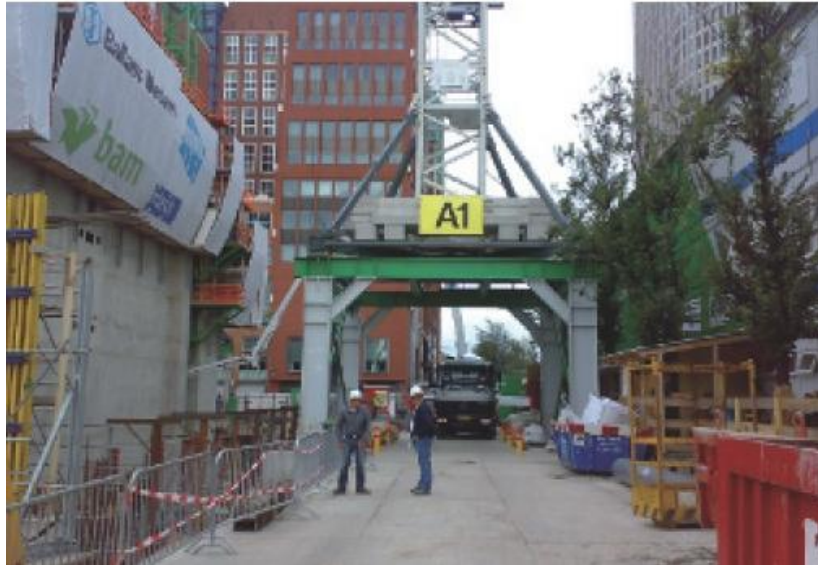
Figure 150 Portal structure for the tower cranes [Herwijnen 2011]
