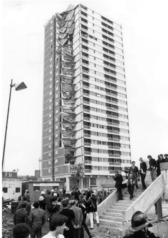
Figure 118 Progressive collapse at the Ronan Point tower [Wikipedia 2012]
