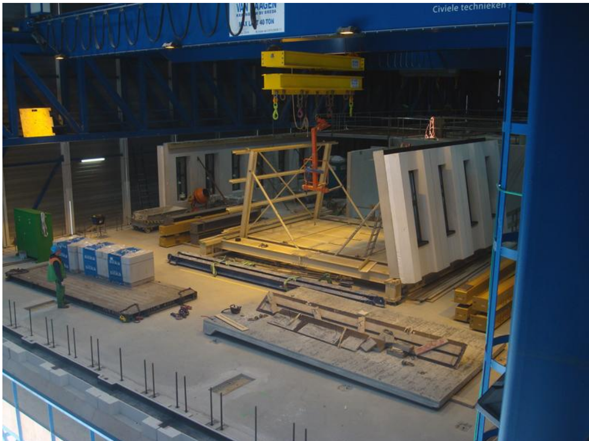
Figure 18 Gantry crane with large stabiliser
