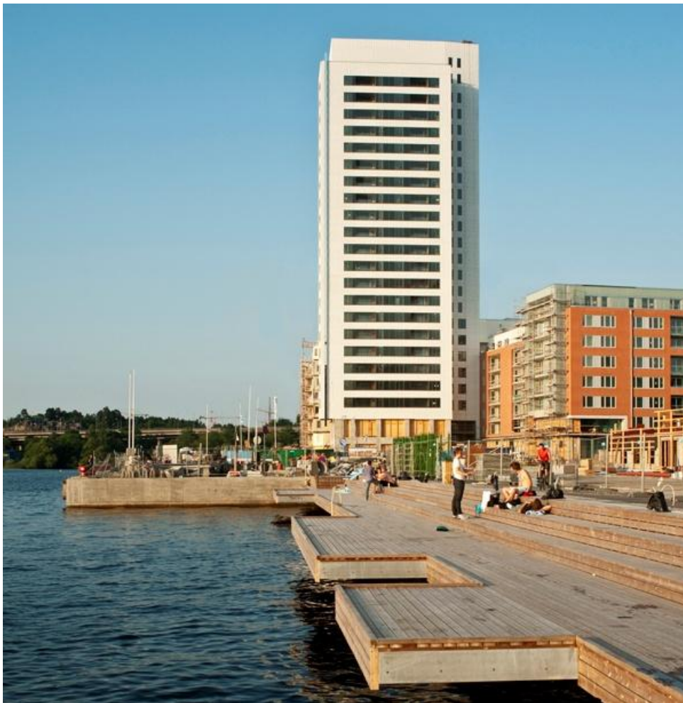
Figure 23 Lindhagskrapan tower in Sweden [Svensk Betong]
