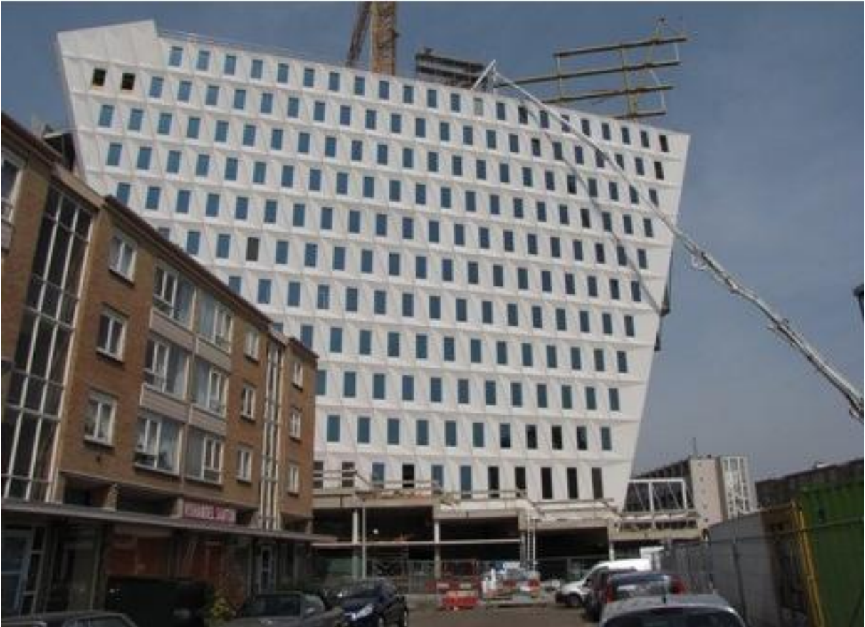
Figure 63 Alternating windows at the Stadskantoor in The Hague [Hurks Delphi Engineering 2012]
