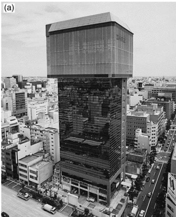
Figure 167 SMART System during Construction [Maeda 1998]
