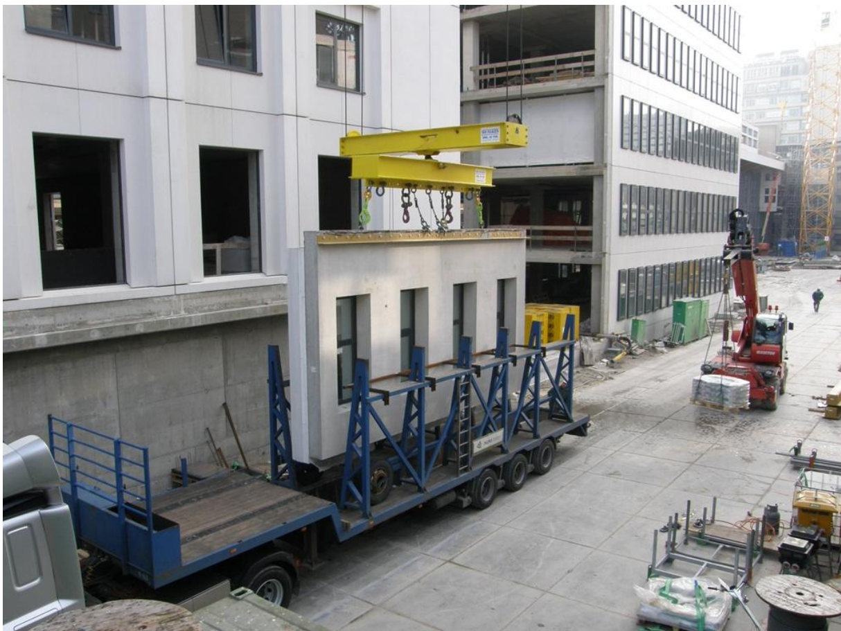
Figure 26 Broad stabiliser with two gantry cranes [Nieuwbouw EMC]
