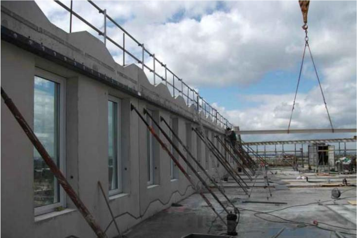
Figure 62 Wet horizontal tooth connection [Hurks Delphi Engineering 2012]
