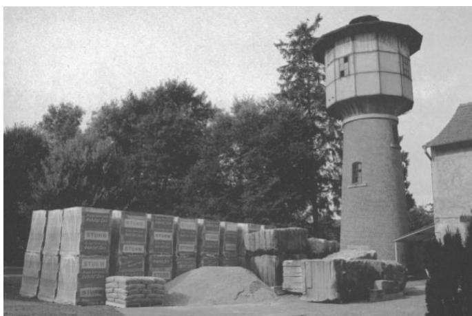
Figure 13: Construction materials displayed near the tower before its demolition.
