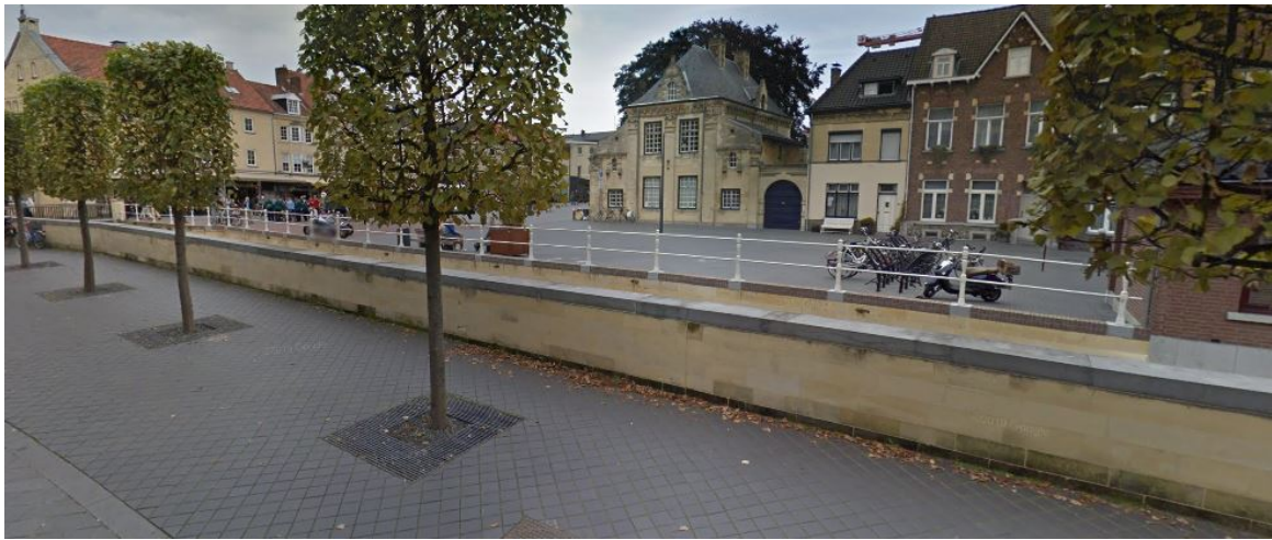
(a) The Bogaardlaan in Valkenburg. Only one side of the river is protected by a quay wall
