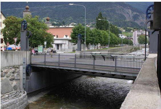
(a) Vertical lift bridge Brig
