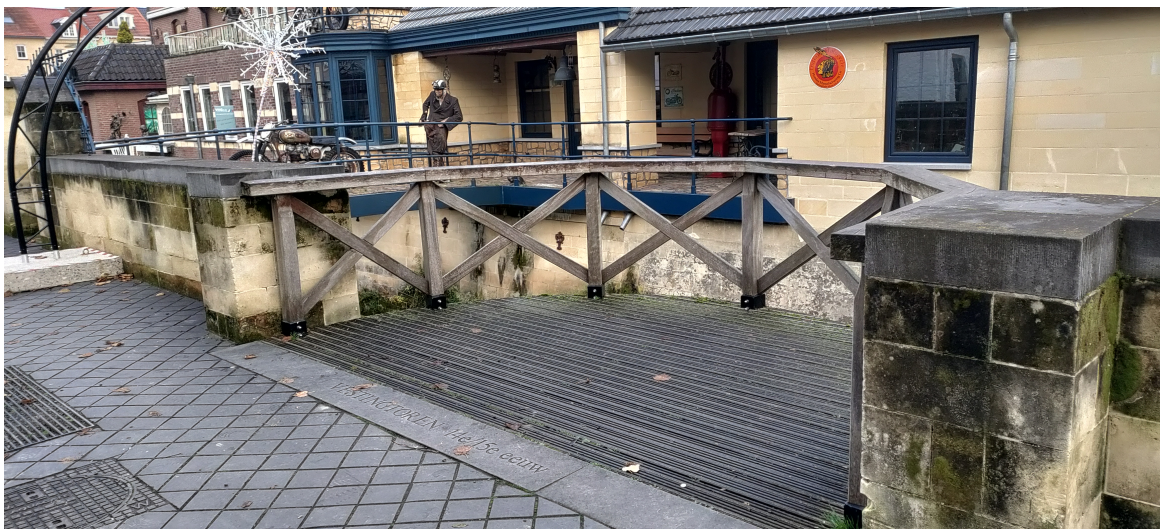
(b) The facade is sometimes incorporated in the quay wall
