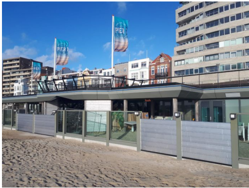
(a) A glass storm flood barrier on the beach in Vlissingen (KWS, n.d.)
