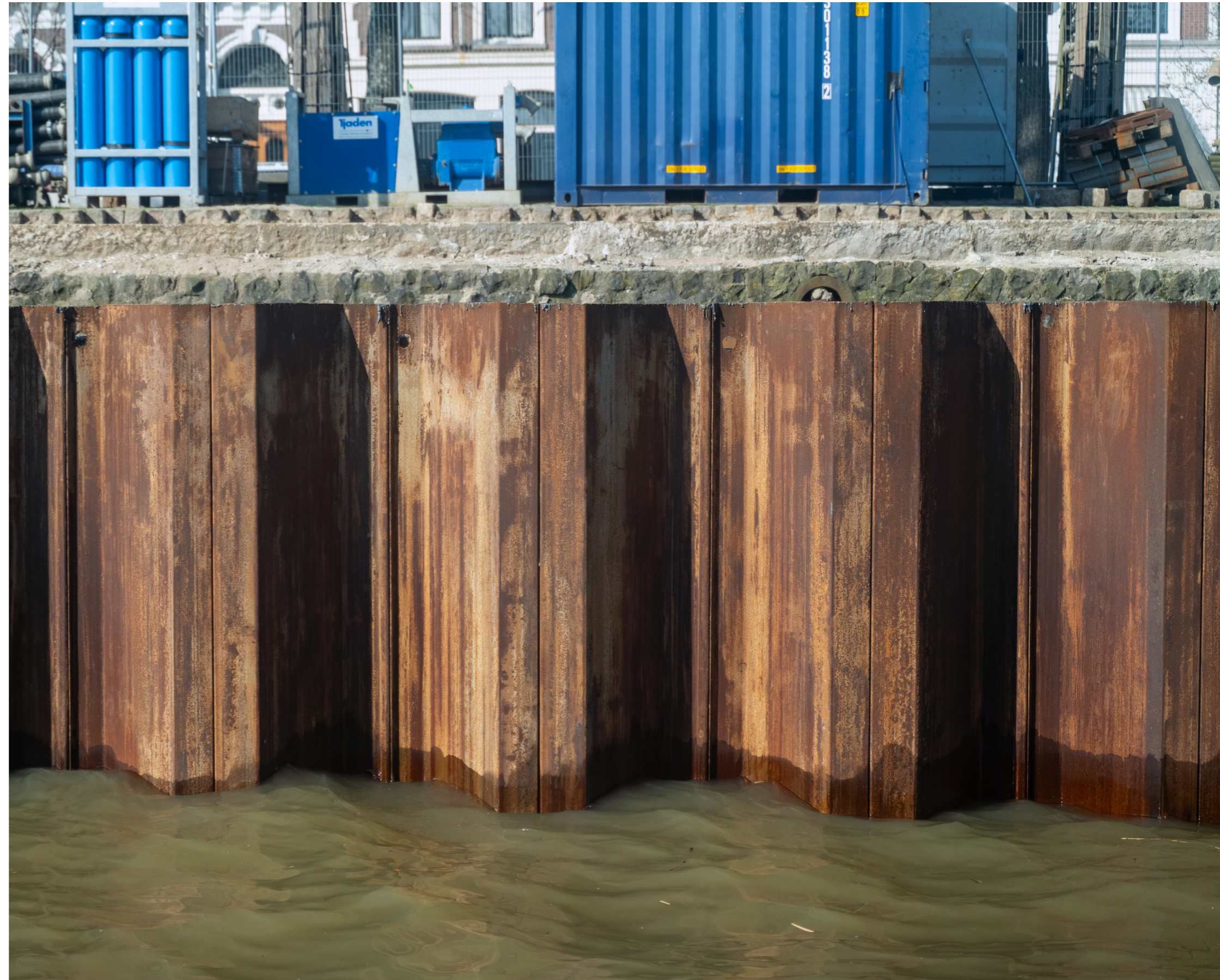
Figure 7 – Metal Sheet Pile Construction
