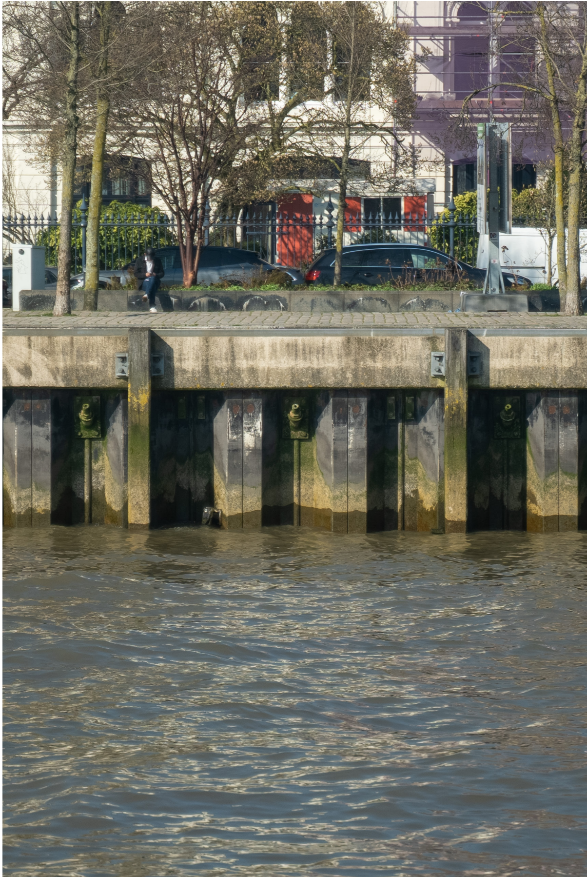
Figure 18 – Anchor Heads
