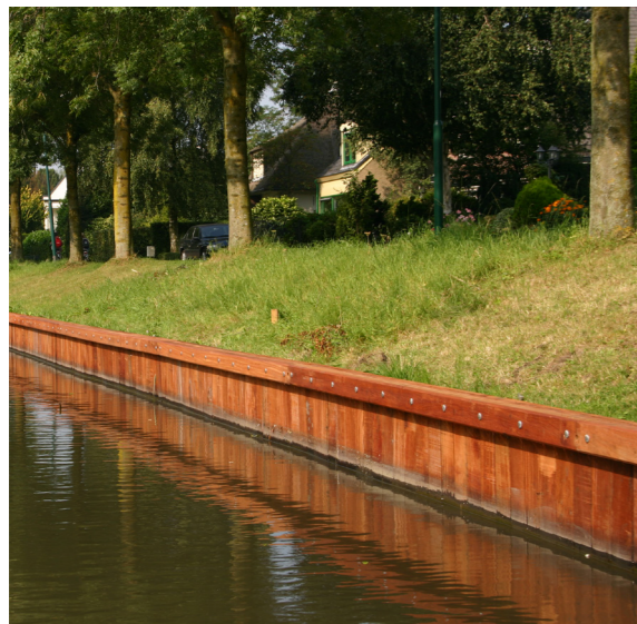
Figure 8 – Wooden Sheet Piles
