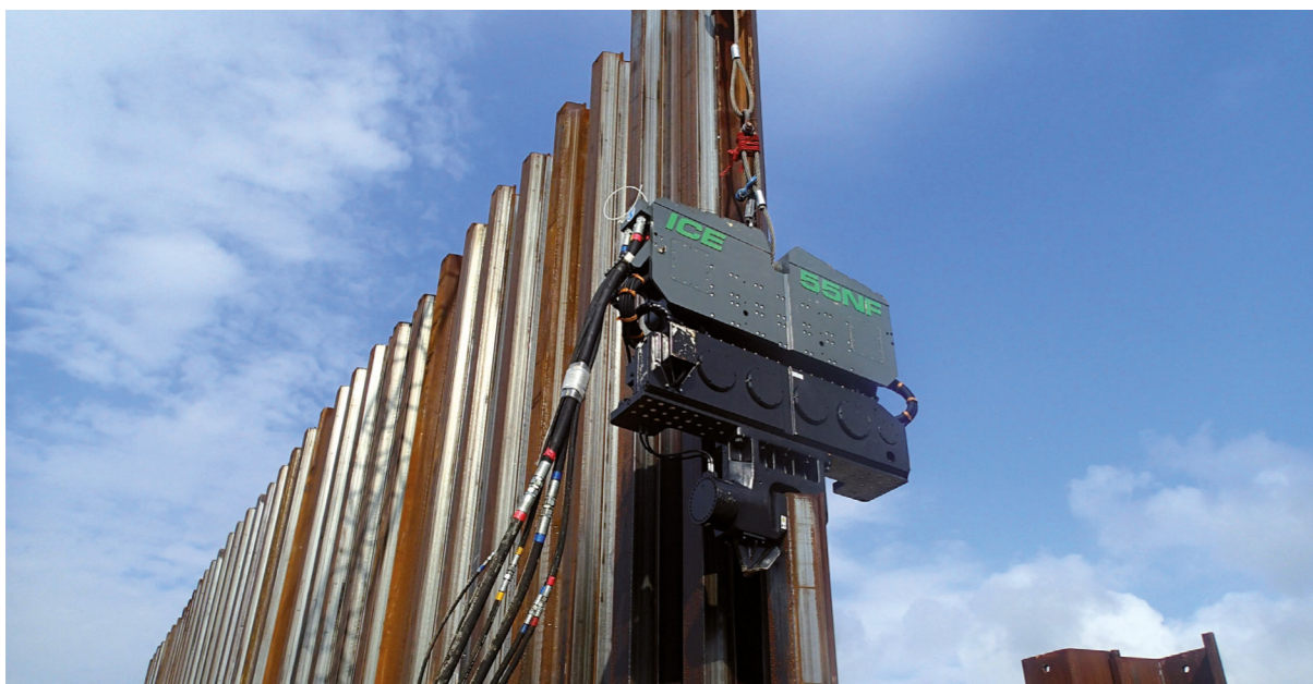
Figure 14 – Vibratory Driving
