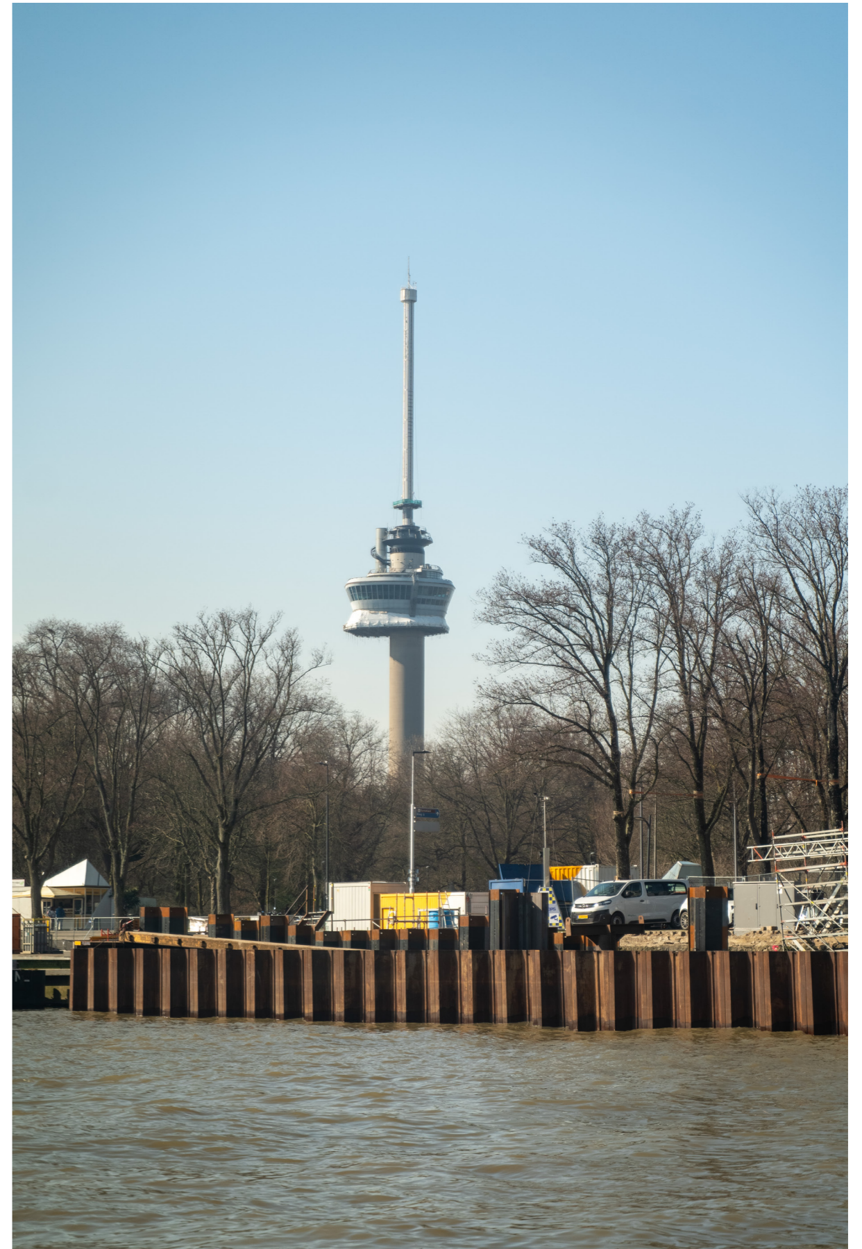
Figure 36 – New sheet piles being installed in Rotterdam
