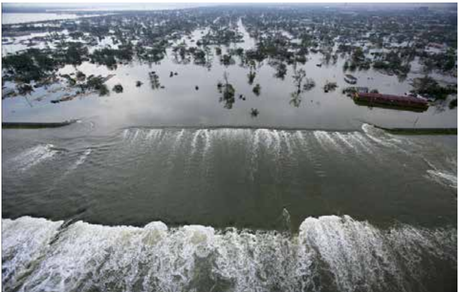
13 New Orleans' Dike Failure © Getty Images
