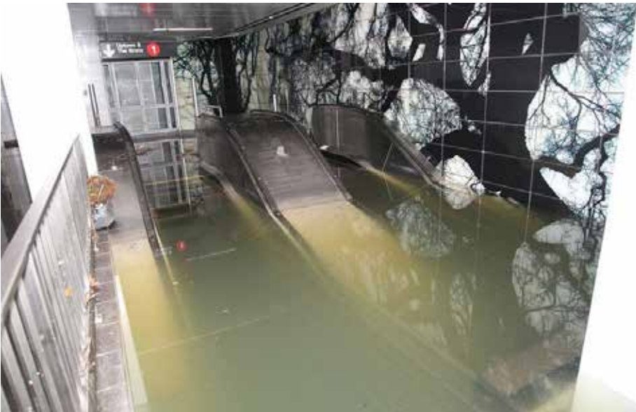
14 Uptown and Bronk Subway Line station flooded during Sandy © CNN
