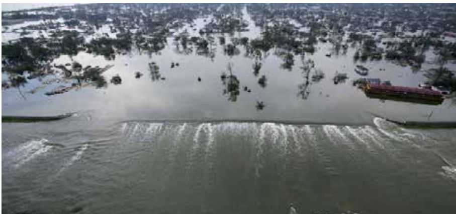
8 New Orleans dike failure during Katrina © CNN
