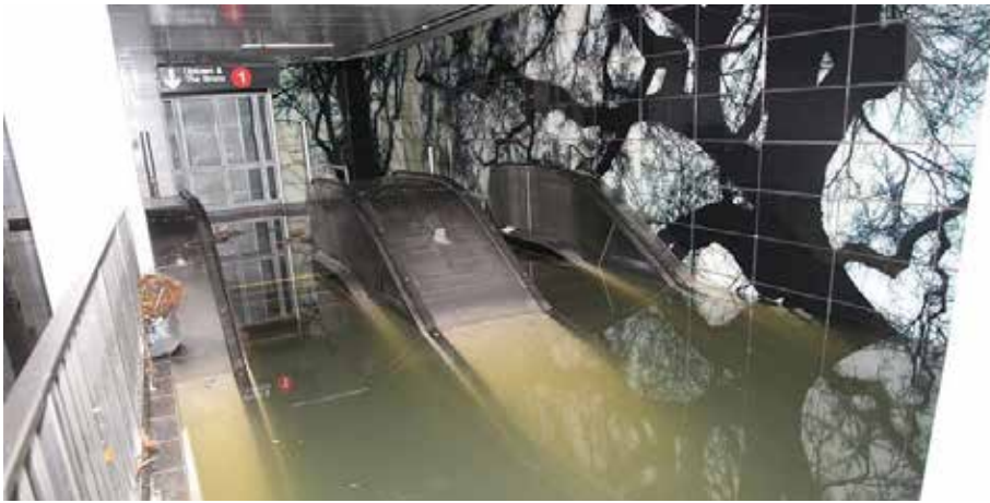
15 Subway station flooded during Sandy © NYC
