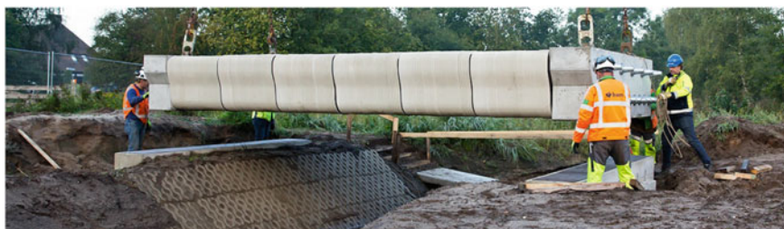
Fig. 6.10 Printed showcase segment for the pedestrian and bicycle bridge (Bos et al. 2019)
