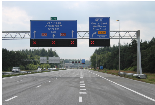
Figure 2.1: Matrix sign portal along the A12 road, retrieved from Rijkswaterstaat image database, 2019
