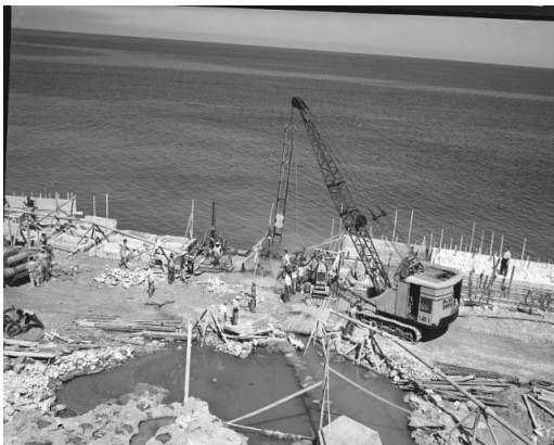
Figure G.4: Construction of the wall in water seen from above
