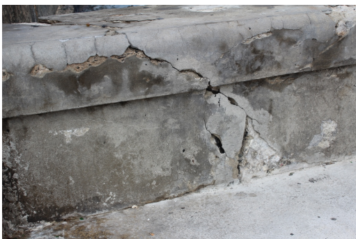
Figure 5.6: Current condition of the wall in section 2 showing cracking
