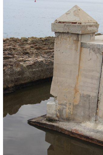
Figure 5.11: Condition of the sea wall in section 4 showing the scour problem
