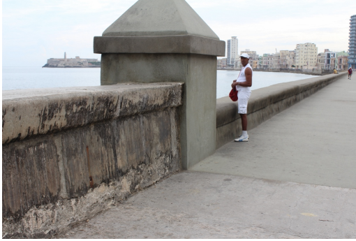
Figure 5.8: Change of crest height between sections 2 and 3
