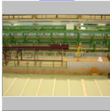
construction of flume side view upstream part.jpg 286.93 KB
