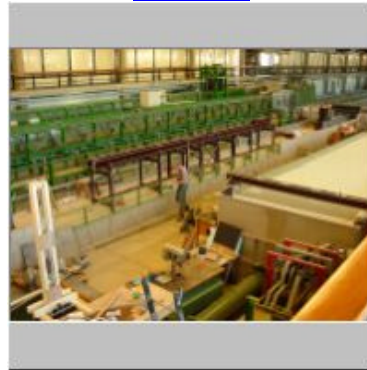
Construction of flume with Jaap complete view 2.jpg 421.77 KB
