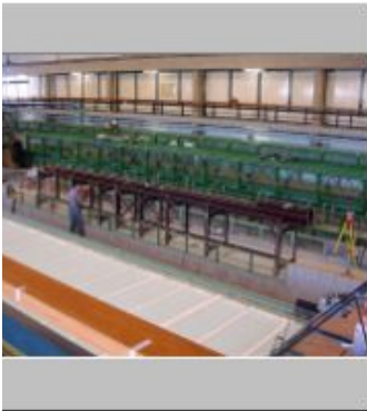
nstruction of flume with Jaap complete view.jpg 358.48 KB
