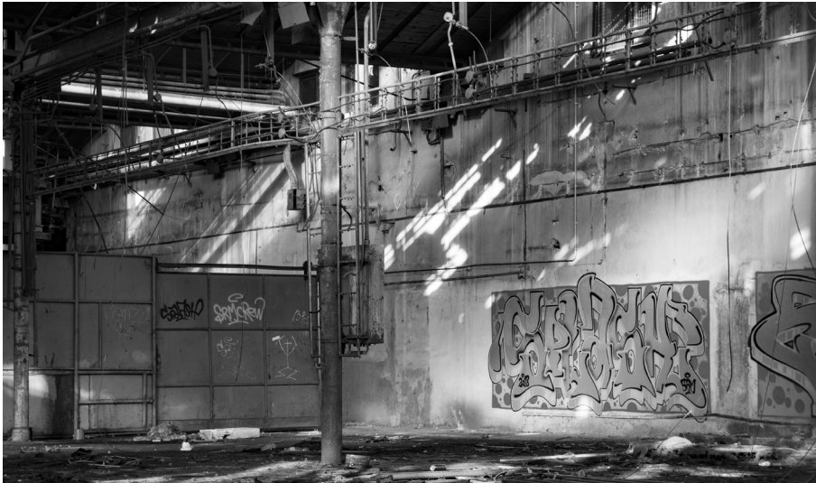
Figure 75: The interior of a building in bad condition
