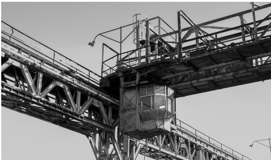
Figure 76: An abandoned industrial crane from Csepel
