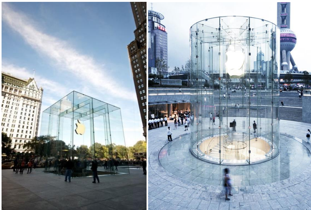
Figure 2 Left: Apple Cube New York, right: Apple IFC Shanghai (both retrieved from https://www.eoengineers.com/en/projects )
