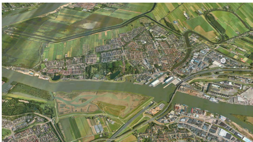
Fig. 3 Alblasserdam riverbanks: 1. Mercon Kloos; 2. Alblasserwerf (former 'De Oude Werf transformed to housing'); 3. OceAnco (former 'van de Giessen de Noord'; 4. Bridge over river Noord; 5. Nedstaal. Photograph Cees van de Wal Fotografie and Film; released under a Creative Commons Attribution-NonCommercial-NoDerivatives 4.0 International License
