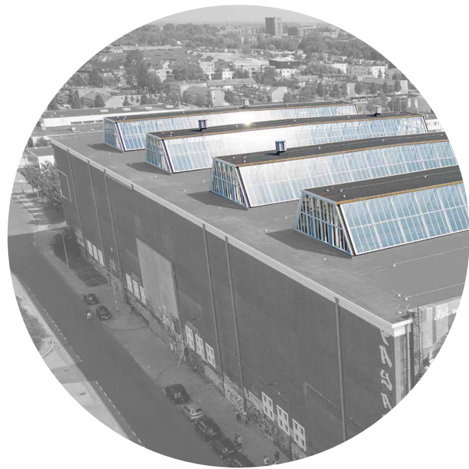
Restored skylights at NDSM wharf
