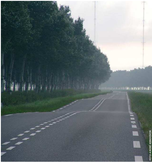
Figure 1.1: Natural speed bumps have appeared in the Vogelweg in Southern Flevoland due to an ancient buried channel deposits made by the river Eem [21].
