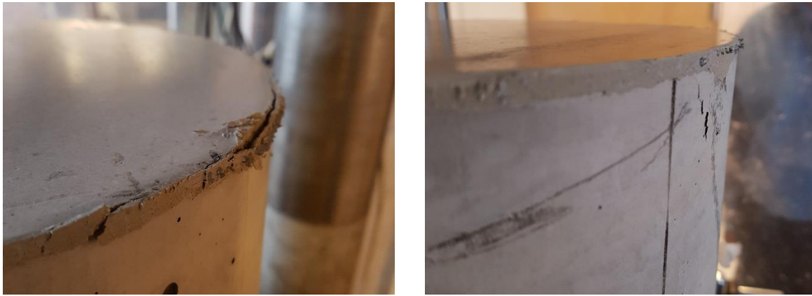
Figure 5.43. Spalling of the cylinder after the test.
