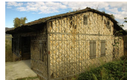
Fig. 20- Wall cell infill system. Image by Hamiyet Özen
