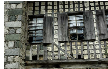
Fig. 19- Wall cell infill system. Image by Hamiyet Özen
