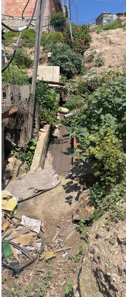
Image by Daniela Diaz- Resident-constructed drainage canal, currently clogged with garbage and characterized by strong odors and mosquito infestations.
