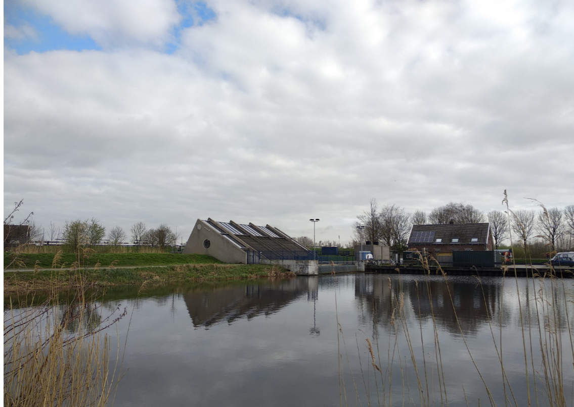
Figure 1.5 - Current Kok pumping station
