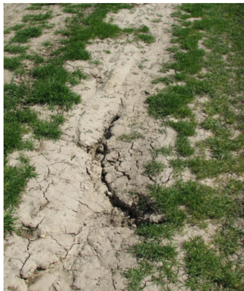
Figure 2. Surface drying crack
