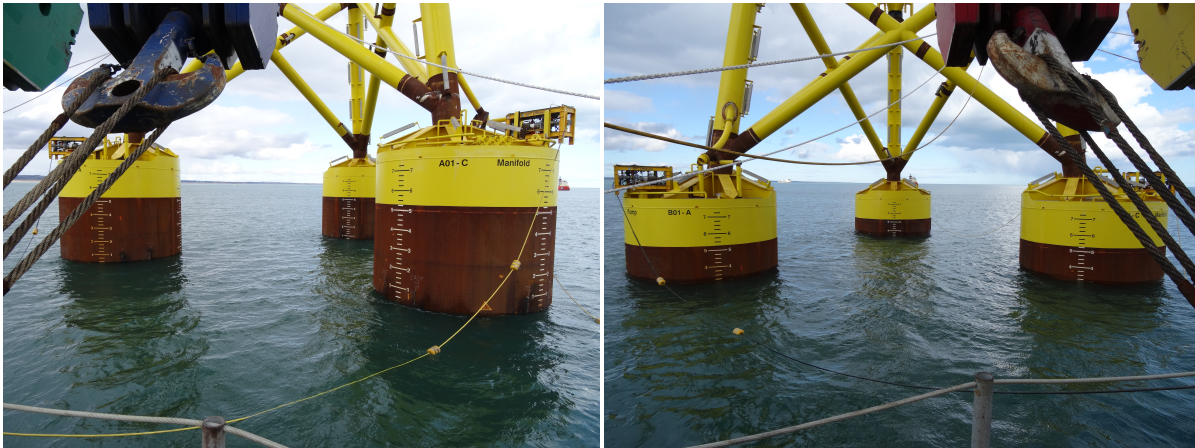
Figure 1.4: Suction Bucket Jacket installation through the splash zone
