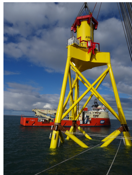
Figure 1.6: Installed SBJ support structure
