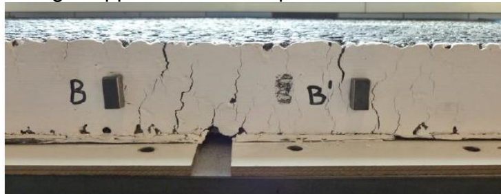
Figure 3: Specimen after cracking in joint-tester at Breijn-Heijmans.
