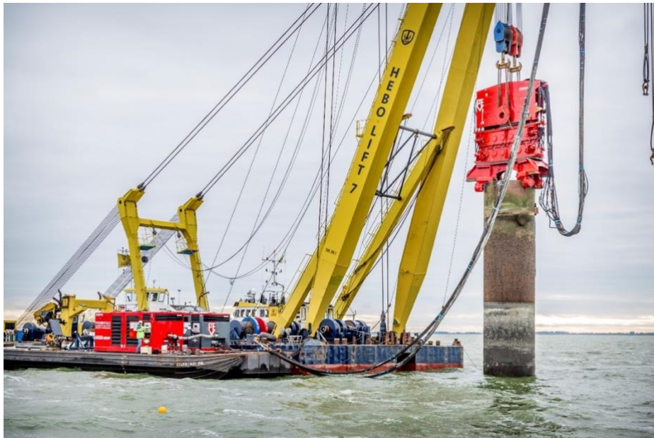
Figure 4.5: Vibratory Lifting Tool removing a monopile at OWF Lely, the Netherlands [Nuon, 2016]
