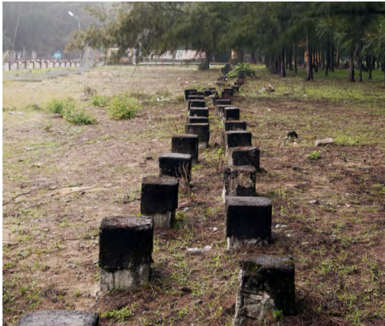
Figure A.9: Pillar heads used to close the Hoa Duan inlet
