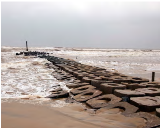
Figure A.7: Groyne on south east side
