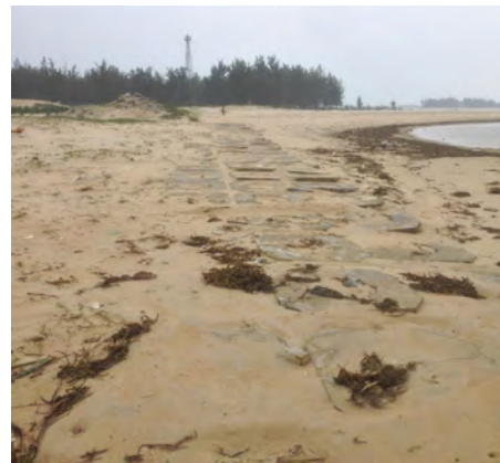
Figure A.8: Part of groyne covered by sediment
