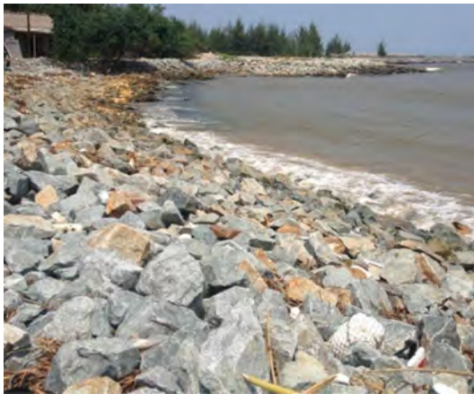
Figure 10.6: Bank protection at Thuan An inlet
