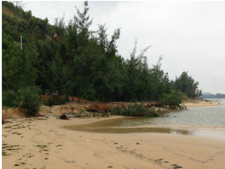
Figure A.33: Erosion at down drift side of Tu Hien inlet
