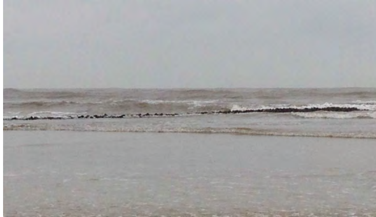
Figure A.30: Groyne near Loc Thuy inlet
