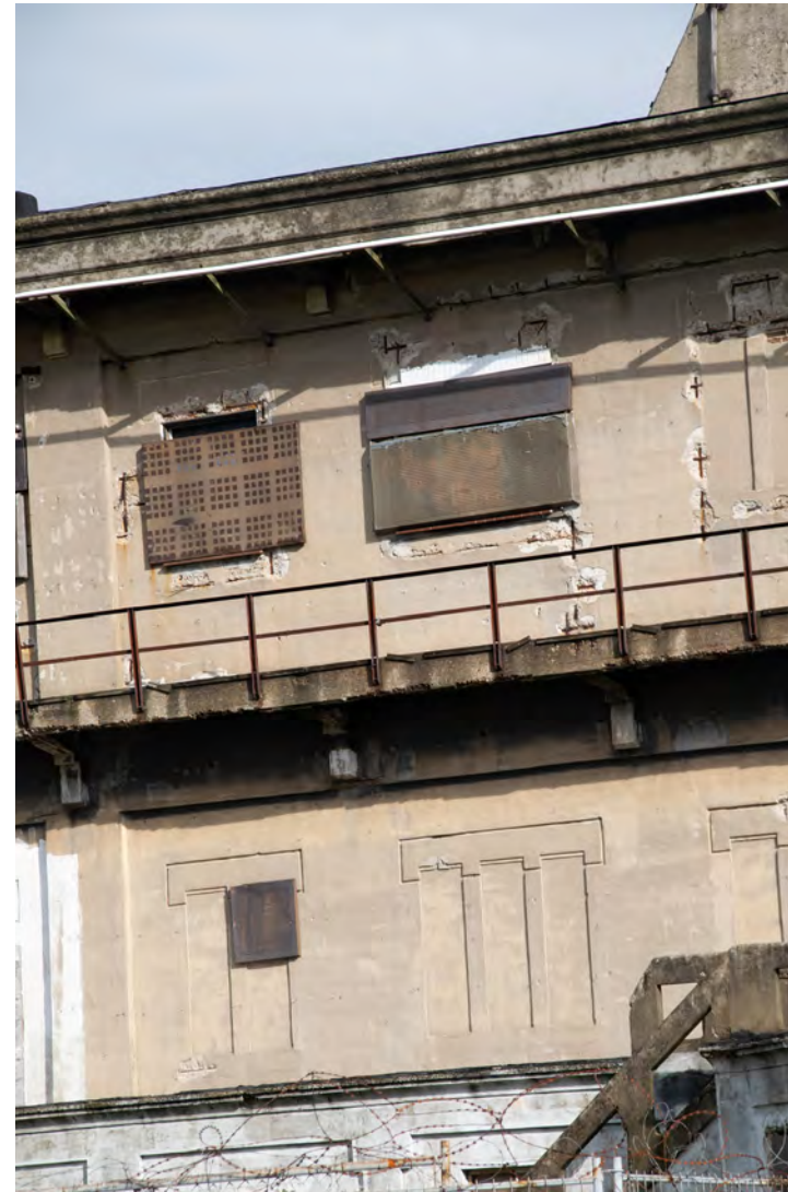
'Kunstzandsteenpleister' rendering on South-West facade
