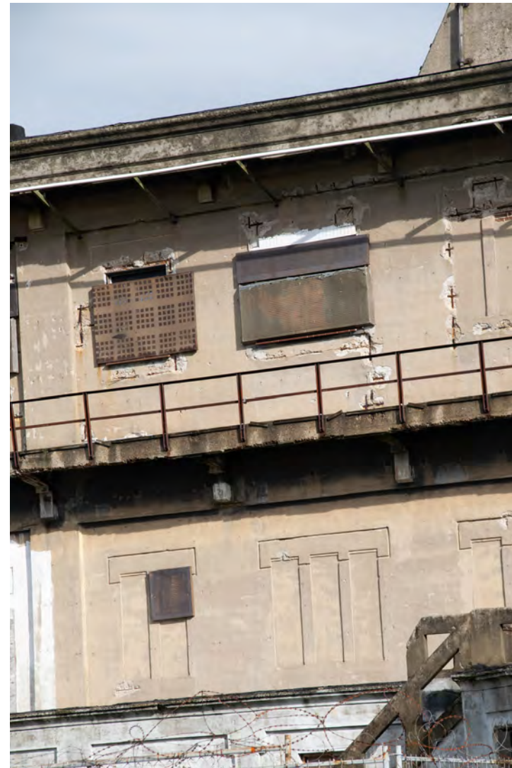
'Kunstzandsteenpleister' rendering on South-West facade
