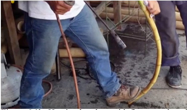
Figure 6.1b: Heating bamboo with flame torch and
