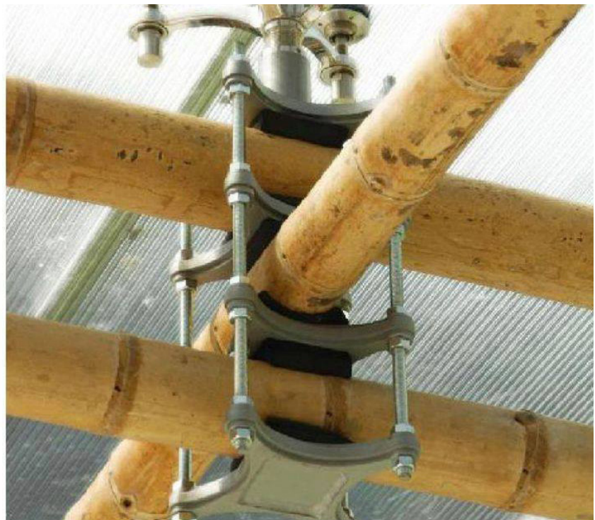
Figure 14.8g: Bamboo x-joint (Val, 2011). Figure 14.8h: Bamboo-bamboo grid connection(unknown).
