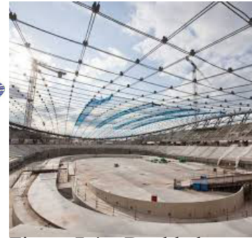
Figure 7.4g: Double layer steel cable grid
