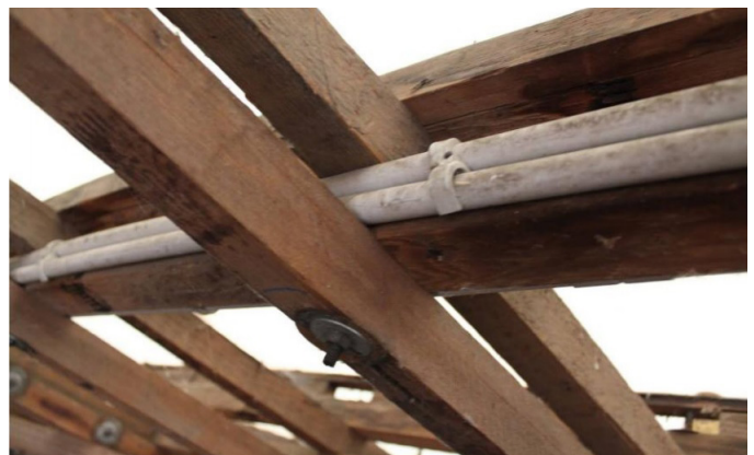
Figure 7.4e: Nodes bolted fixing
