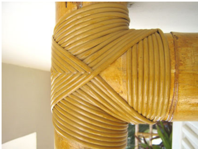
Figure 5.1a: Lashing joint using bamboo cane rope.
