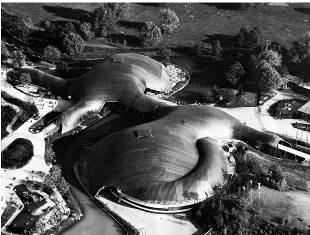
Figure 7.4b: Aerial View Mannheim Multihalle
