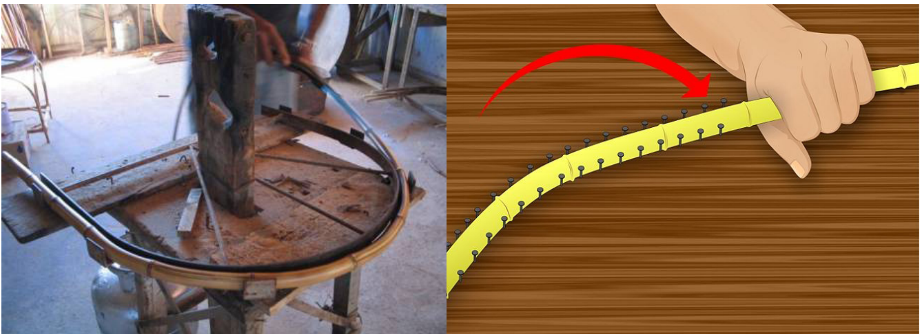
Figure 6.1a: Formwork of bamboo using wood plugs and nails
