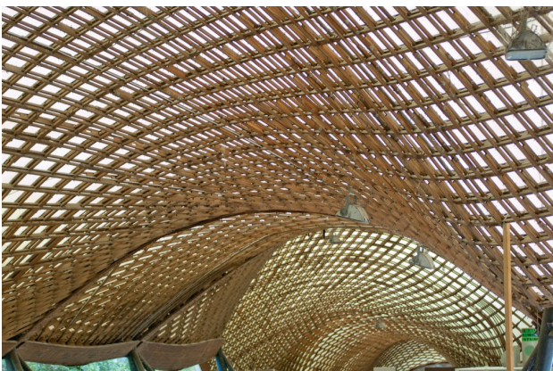
Figure 7.4d: Free form shell of Mannheim Multihalle
