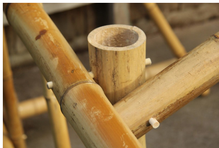
Figure 5.1e: Wooden dowels passed through slotted bamboo
