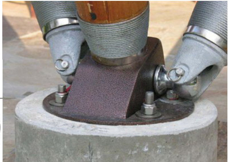
Figure 14.8c: Bamboo end connection. ref: (unknown)
