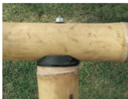
Figure 5.1r: Connection using rubber end supports, Adan Piza
