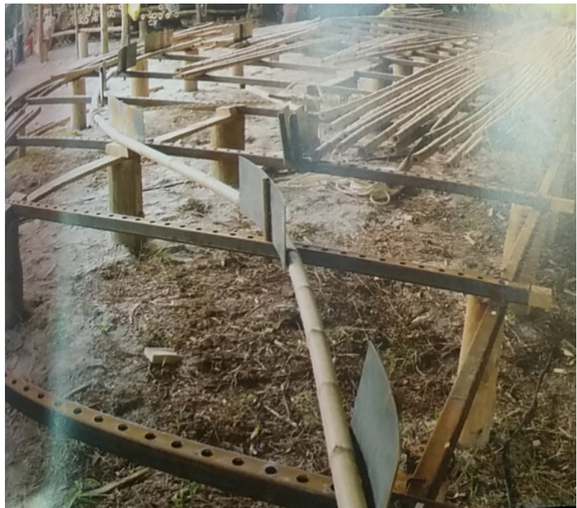
Figure 11.4e: Bamboo bending using grid layout ref: 24H Architect
