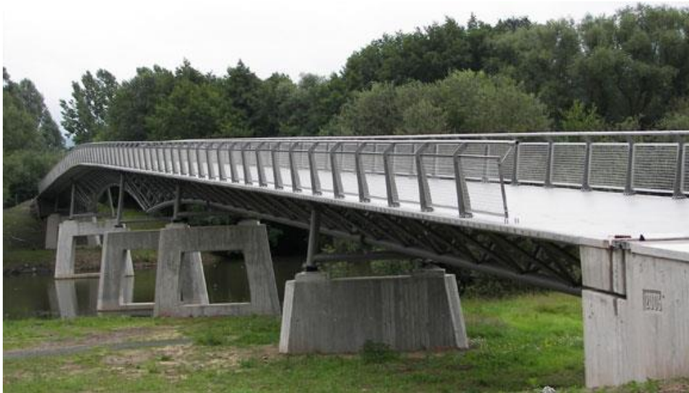
Figure 22: The 'Gärtnerplatzbrücke' pedestrian bridge
