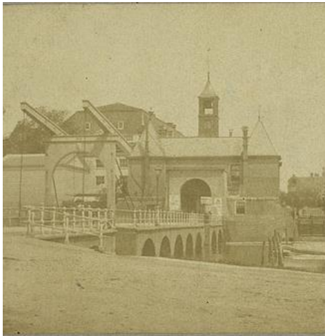
Figure 2-2: Old Leiden bridge, with in background the Leiden Gate
