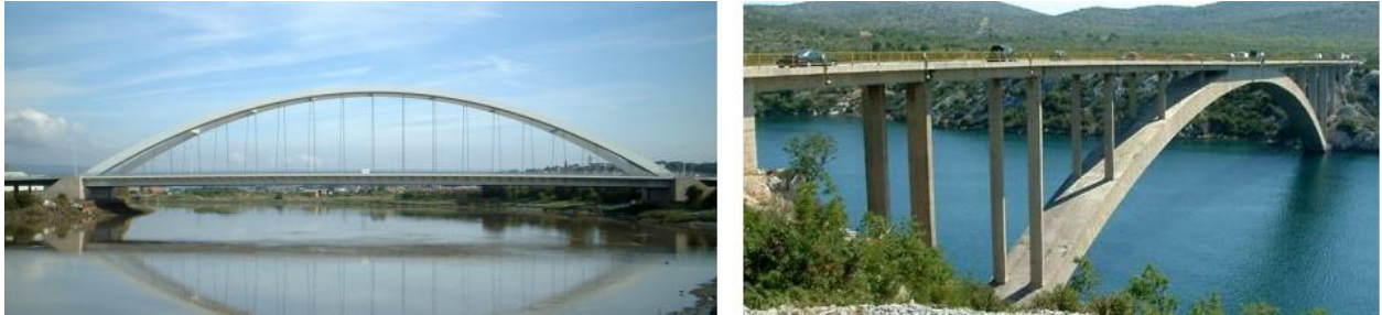
Figure 36: Left: Suspended deck arch bridge; right: Supported deck arch bridge
