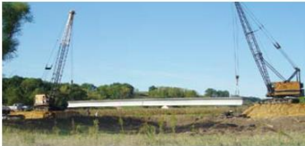
Figure 17: Hoisting of beams
