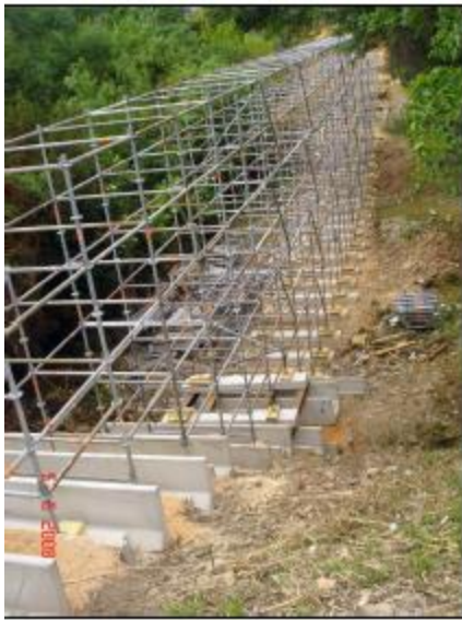
Figure 27: Placing of scaffolding
