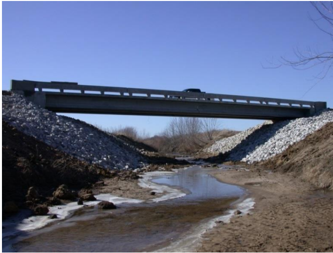
Figure 16: Mars Hill Bridge
