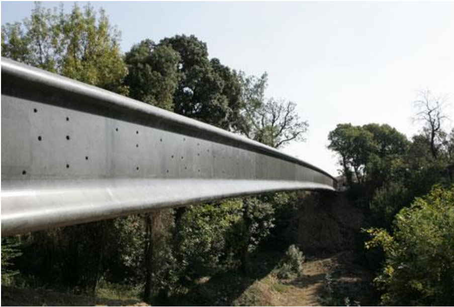
Figure 25: La Passerelle des Anges Footbridge
