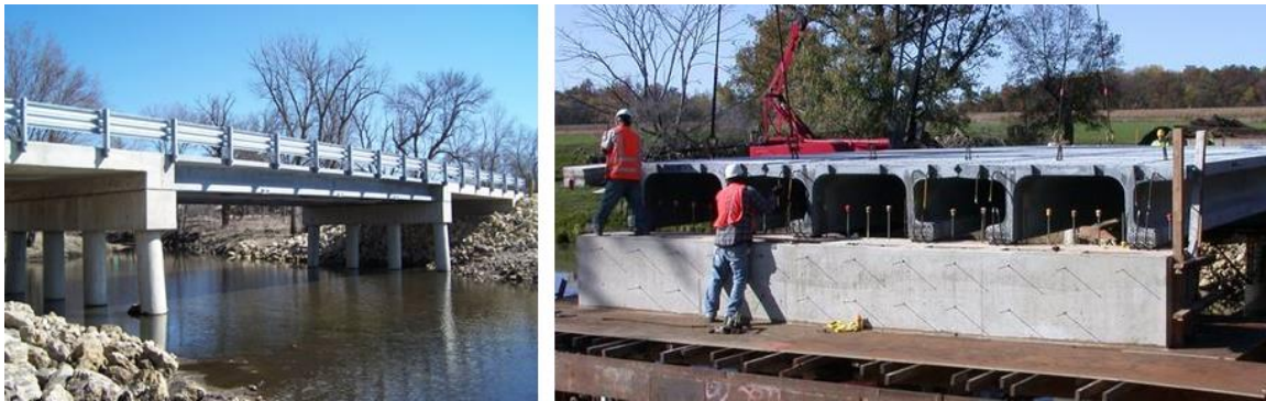
Figure 19: Completed Jakway Park bridge (left) and Erection of the bridge (right).
