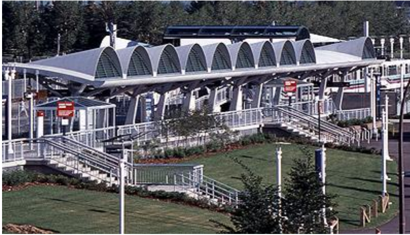
Figure 7: LRT Station Canopy
