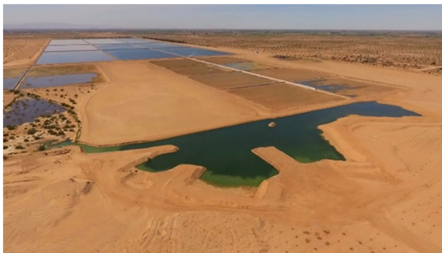
Fig. 8 At San Luis Río Colorado, Sonora, Mexico, oxidation lagoons (at a wastewater treatment plant in the background), have annually discharged 8.2 Mm 3 treated water to intermittent infiltration basins (located at a distance in the middle of the photo) for more than 10 years, and in the foreground some water is starting to be used to
