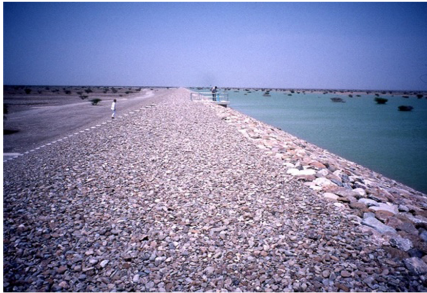
Fig. 6 Ahin recharge dam on the Batinah Plain, Oman, constructed in 1994, is a large dam (crest length 5,640 m, crest height 8 m) with a detention capacity of 6.8 Mm 3 . This is one of the 43 recharge dams, with an aggregated capacity of 95 Mm 3 constructed in Oman during the period 1985–2011 (Oman MRMR 2012). Their purpose is to enhance aquifer recharge primarily to support irrigation; and also to protect the
