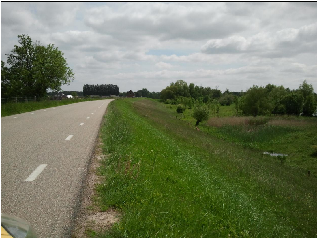
Figure B-26: Photo 10, East end of the Grebbedijk, Hoornwerk
